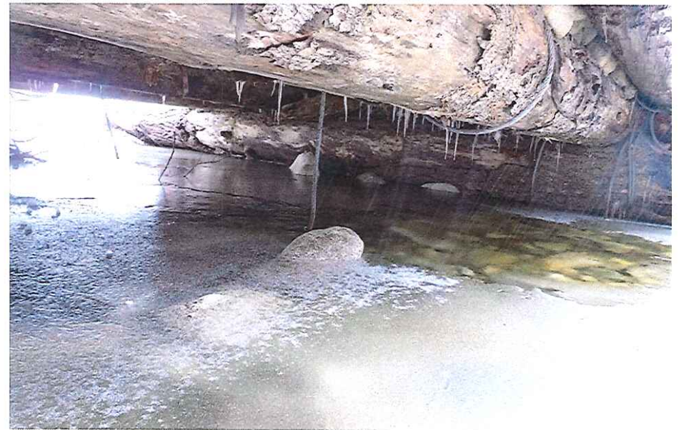
CK2210 Left Abutment
